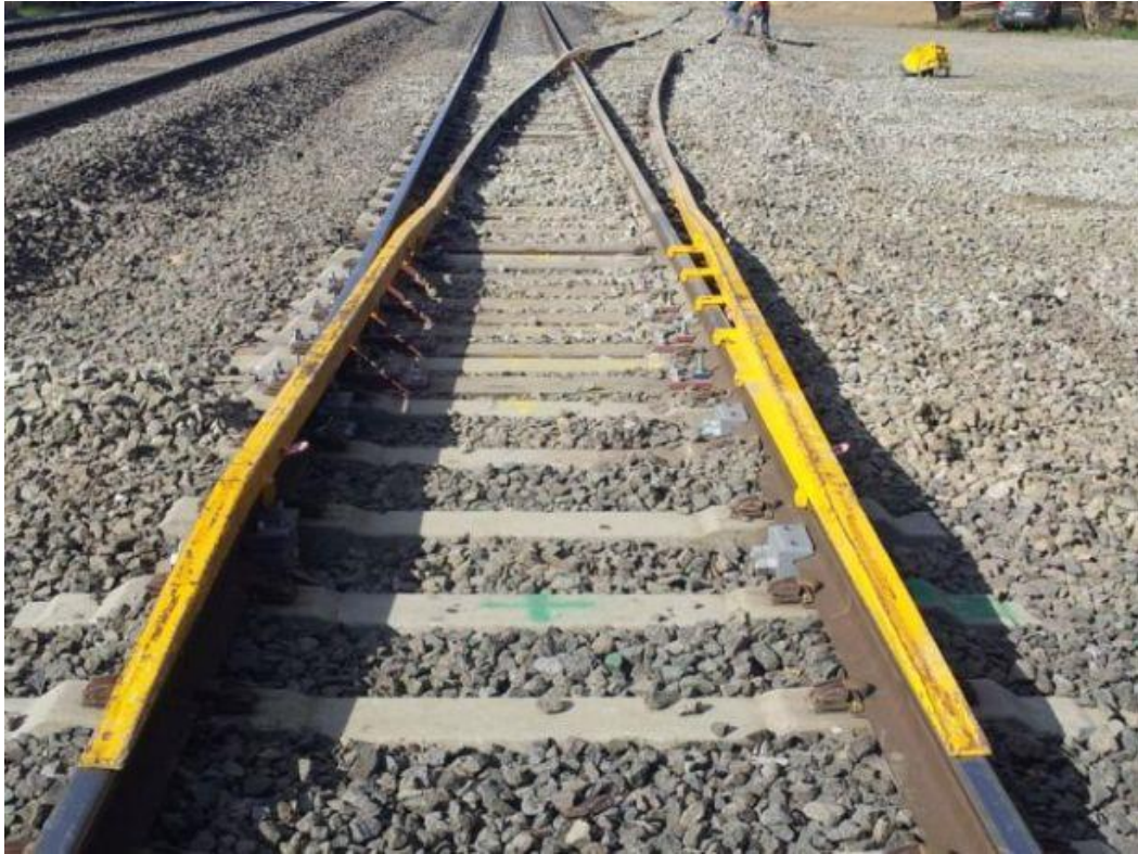
Figure 3.9 Concept F: A temporary over running rail switch. (Credit: Martinus Rail Australia)
