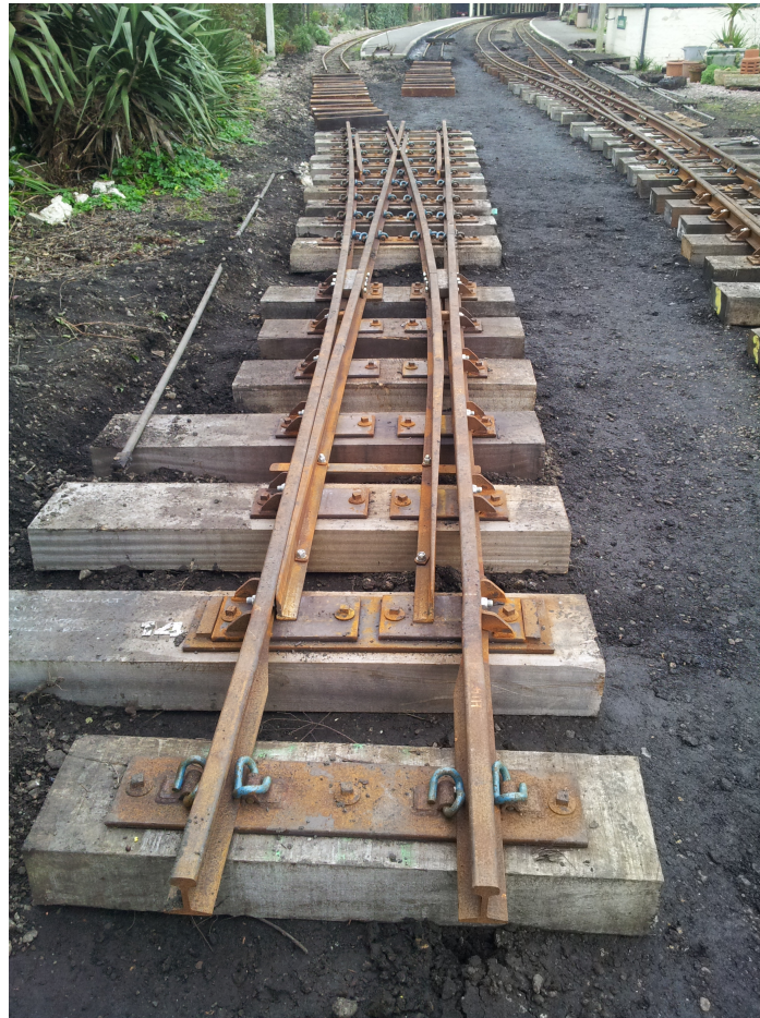
Figure 1.1 A Switch Panel ready for installation as part of remodelling works on the Romney, Hythe and Dymchurch Railway, Kent, England. Though 381mm gauge, all essential components have been scaled down faithfully. Credit: Author
