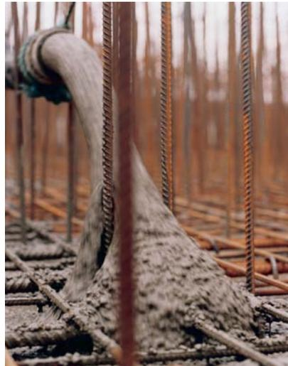
Figure 1. SCC in action (courtesy of Lafarge)
