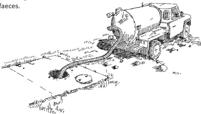
**Figure 12.** Sludge removal
