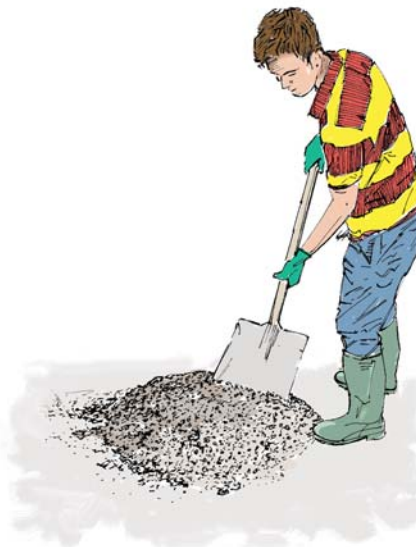
Figure 20. By far the most durable material for an apron slab is good quality concrete
