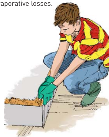
Figure 20. Building a clay dam to hold the curing water on the slab
