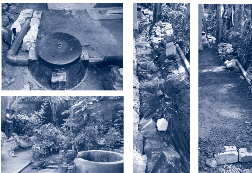
Picture 11_17 to 11_20: Construction of a French-drain filter, connecting a plastic septic tank with a plant-bed
