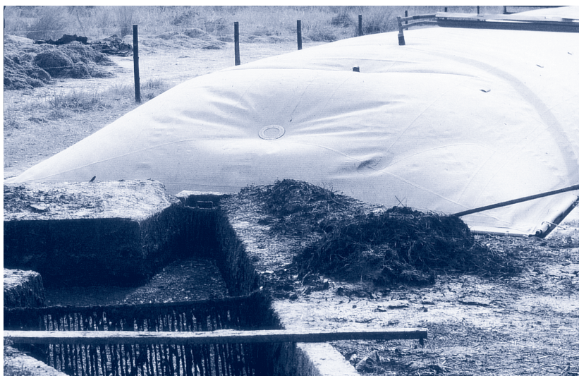
Picture 11_50: Tent gas storage above a liquid ma- nure tank. Biogas plant constructed by SODEPRA and GTZ at a cattle park in Ferkessedougou, Ivory Coast.
