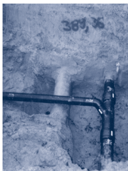
Picture 11_29 to 11_31: PE-HD vacuum Pipe with individual connection (left), collection chamber (centre), waste- water collection, water supply and stormwater-drai- nage pipes in one trench (right)
