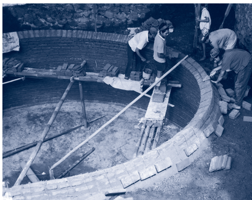
Picture 11_48: Fixed-dome bio-gas plant for cattle dung, under construction by CYSD and BORDA at a farm in Orissa, India
