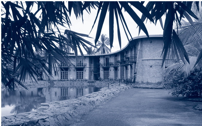
Picture 7.8: DEWATS at a hotel in Cochin, India; large-size ponds are used for post- treatment
