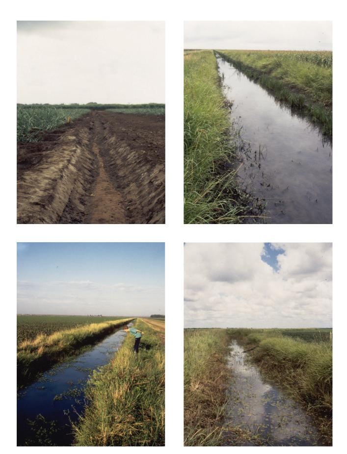
Plate 3.2 Cycle of aquatic weed growth in an irrigation channel following maintenance (see Figure 3.3)
