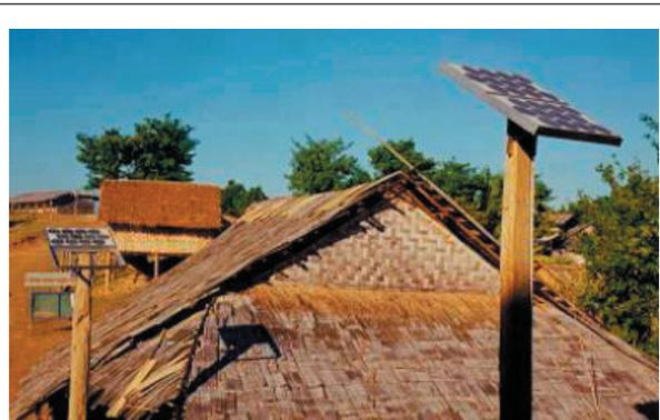
**Photo 2. Solar home systems are popular in Laos. Sizes available under the MIH program are 20W, 30W, 40W and 50W.**
