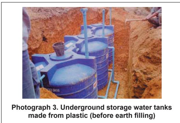
sand and gravel, plastic underground tanks represent an interesting alternative. Several units (unit size up to 2500 liters for transportation matters) can be assembled to reach the total required volume as shown in Photograph 3 and Figure 1.
