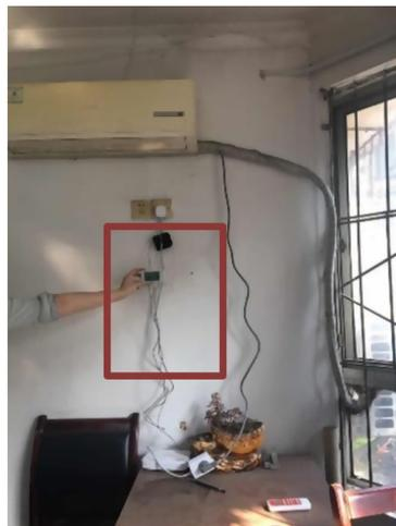
Figure 4-13: Location of the clamp meter to measure AC electricity consumption (source: Yao, 2017).
